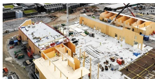
Construction of the EcoDataCenter in Falun using CLT
