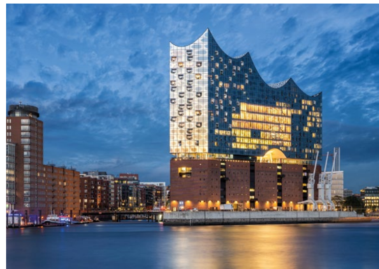
Resting on springs – the Elbphilharmonie concert hall in Hamburg
